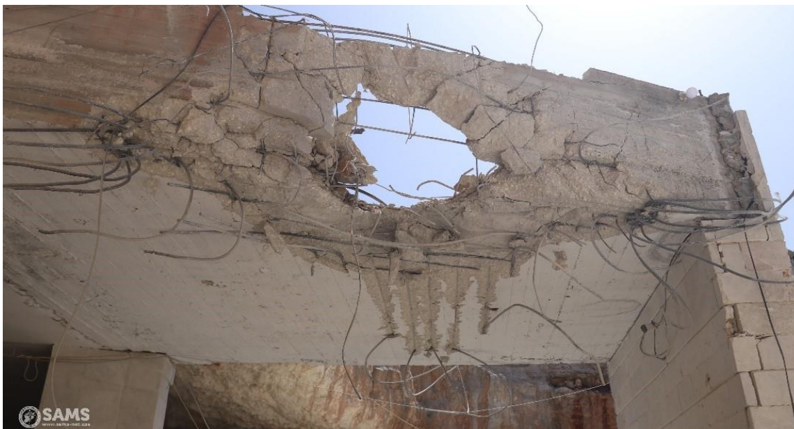
A hole in the ceiling at the front gate of al-Atareb hospital caused by a shell fired during the March 2021 attack. Photo: SAMS
